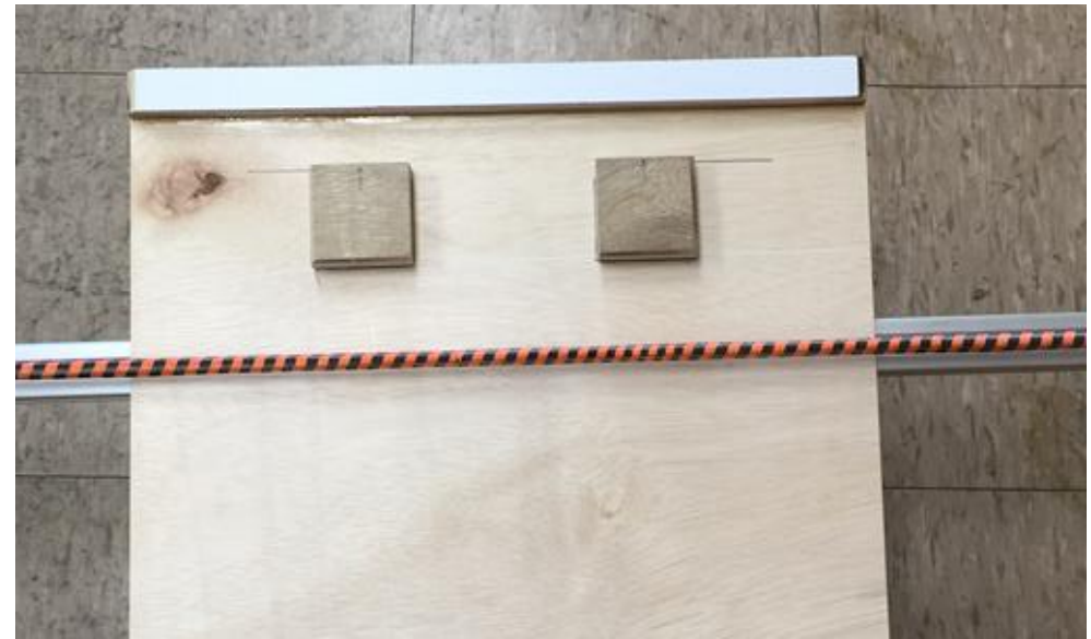
Wooden portion construction
